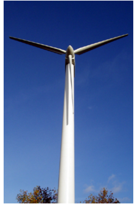
Renewable energy generation
